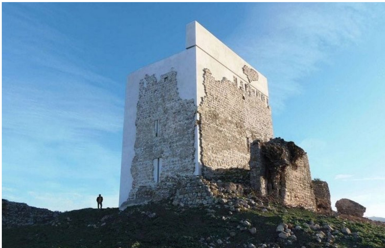
Ил. 2. Замок Матрепа после реставрации ( http://arte-development.com ) Fg. 2. Matrepa Castle after restoration ( http://arte-development.com )
